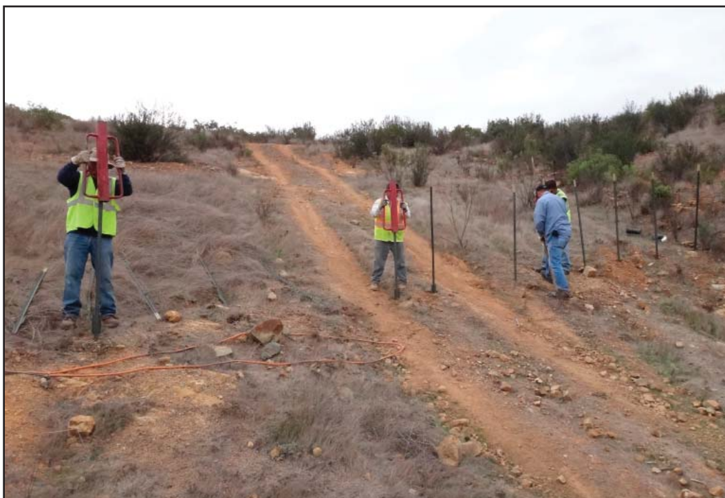
PHOTOGRAPH 2 RECON Crew Installing Fence Posts to Prevent Vehicle Damage to Quino Checkerspot Butterfly Habitat on San Ysidro Parcel
