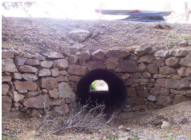
Figure 53. Pipe culvert on SR-78 in Banner Canyon.
