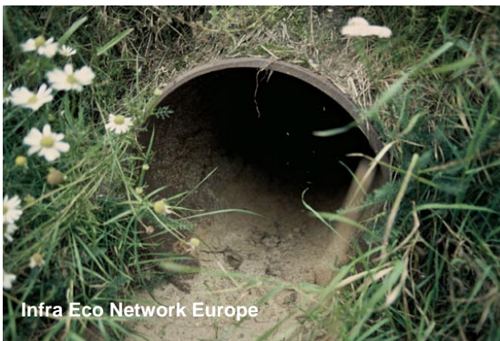
Figure 43. Pipe culvert designed to accommodate small mammals.
