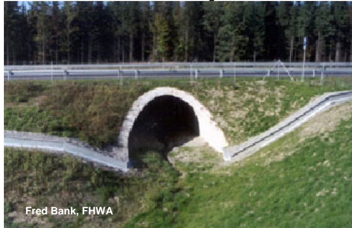
Figure 42. Arched culvert on German highway, with rail for amphibians and fence for larger animals.
