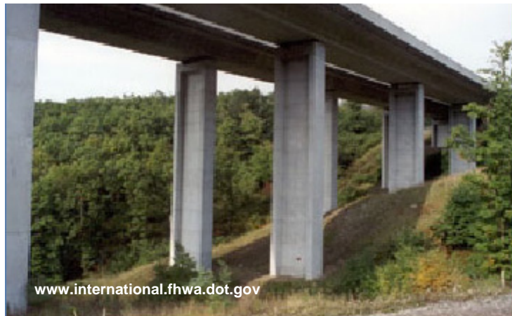
Figure 41. A viaduct in Slovenia built to accommodate wildlife, hydrology, and human connectivity.
