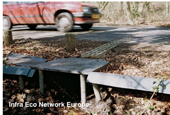
Figure 44. Amphibian tunnels allow light and moisture into the structure.
