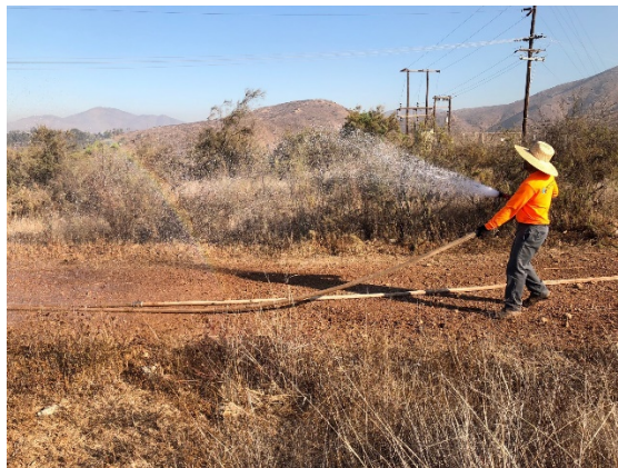
Photo 6. Watering Seed into Road Surface Following Seeding (12/2017)
