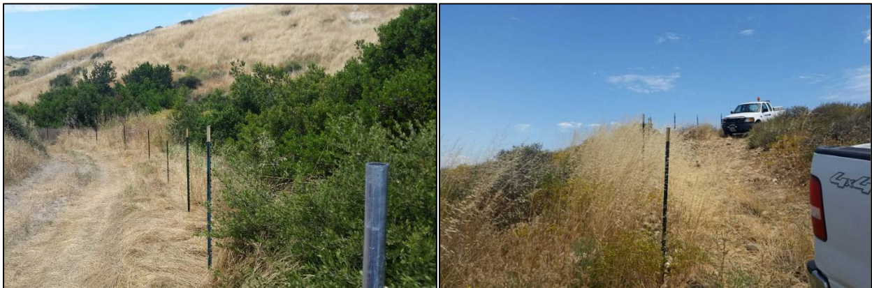
Photos 1 and 2: Fence of being installed along edge of access trail. Wire had not been put on yet. Date taken: 6/6/17.
