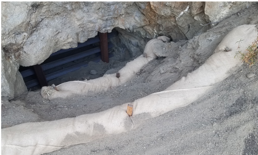
Photo 1. Erosion control materials installed at the entrance of mine ( photo courtesy of RECON Envr. )
