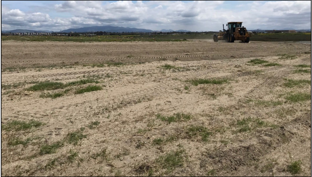
Figure 8. A motor grader scrapes and removes vegetation (San Diego Unified Port District, photo taken on April 3, 2019).
