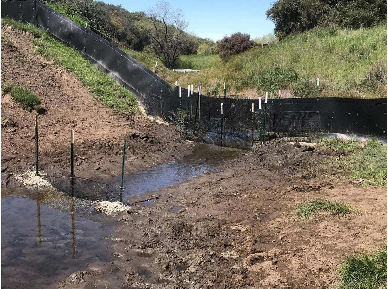
Figure 18. Barrier fencing that is used to reduce the amount of NAS from entering the main pond at TNC Wheatley Preserve on Scholder Creek. The fencing is close to the property boundary. Photograph by Chris Brown.
