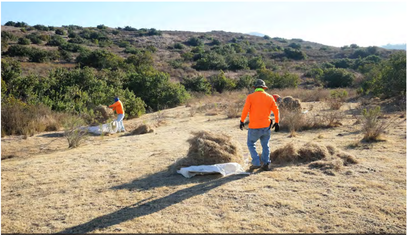
Photo 1: Site 3 Crew Removing Debris Date 12.20.23
