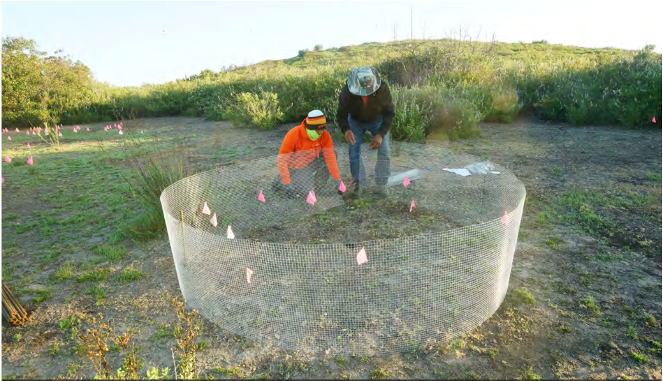
Photo 21: Site 1 Crew Installing Protective Fencing Date 5.7.24
