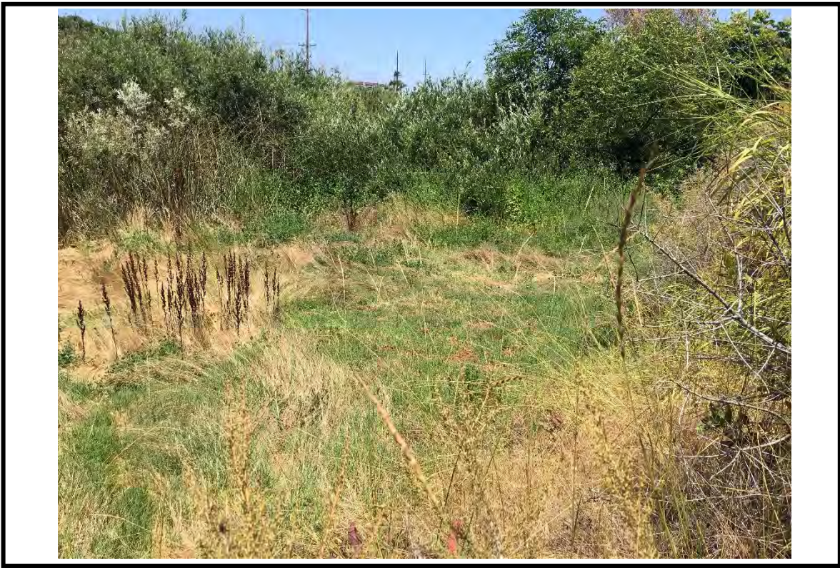
Photo Point 3. View of sediment filled basin Pond 1. Photo date: 7/27/23. Direction: northwest.
