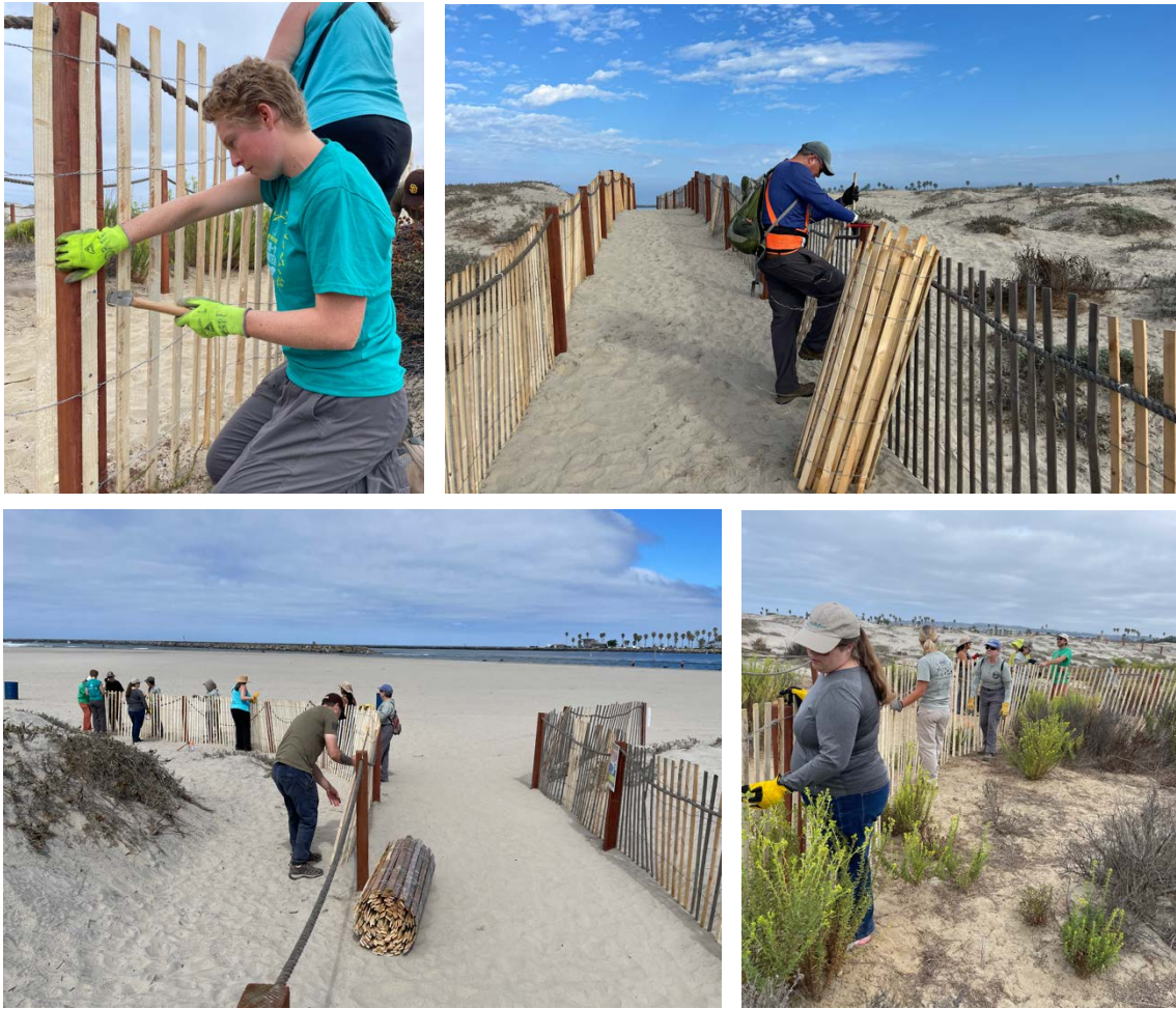
Photo 11-14: New fencing was installed, extended, and repaired by volunteers
